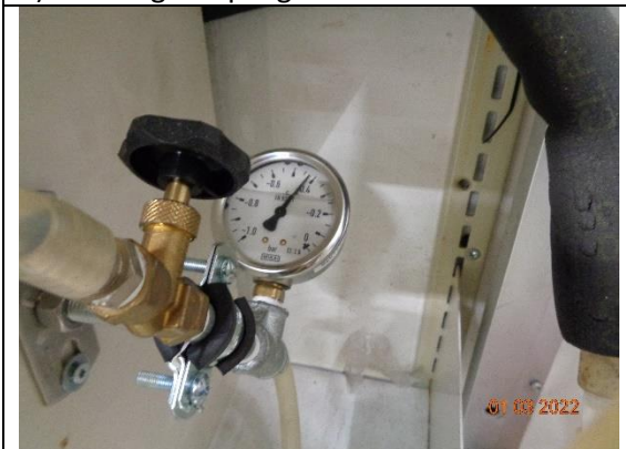
3) Vacuum gauge during leak check
