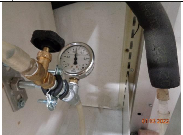
12) Vacuum gauge during leak check
