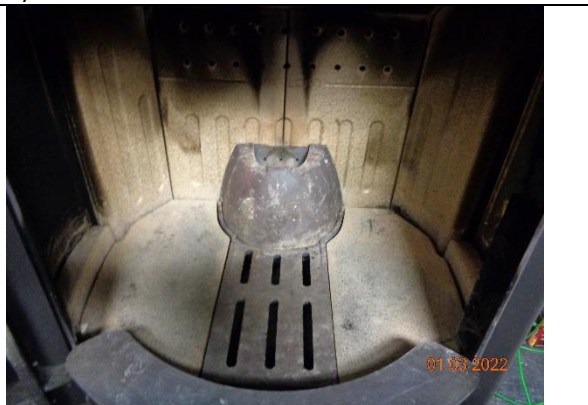
4) Firebox incl pellets burn pot
